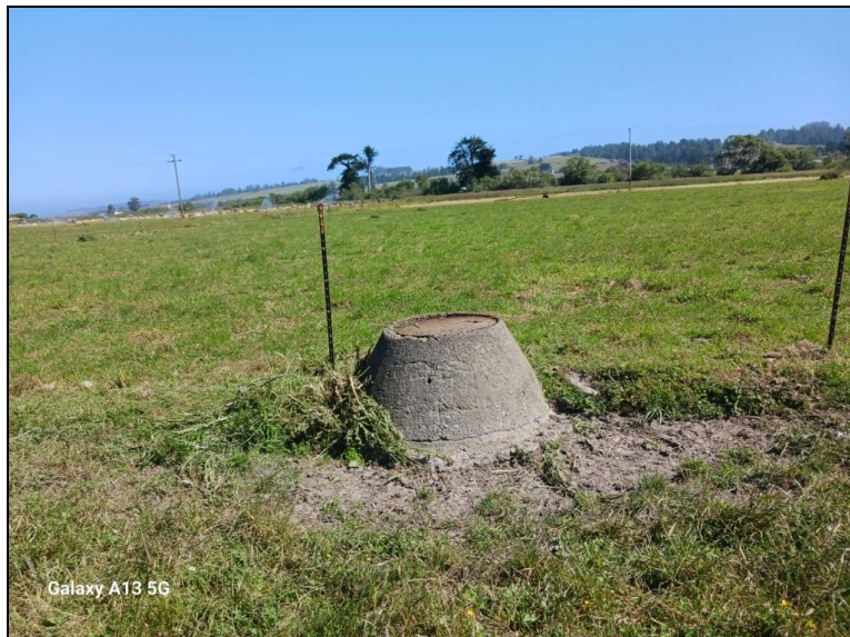
Figure 10 – Existing Wastewater Discharge Pipe Manhole Cover
