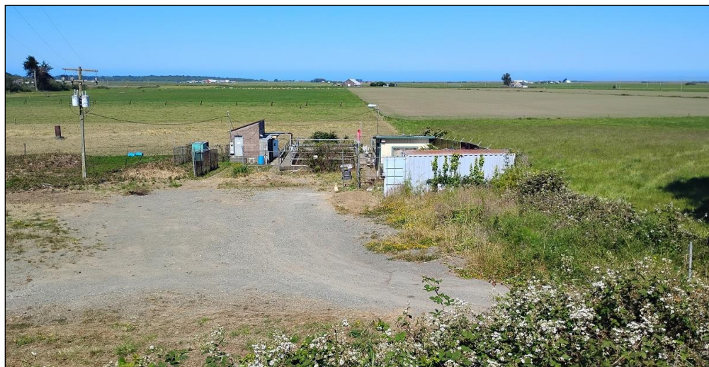
Figure 7 – Existing WWTF Facing West from Eel River Drive
